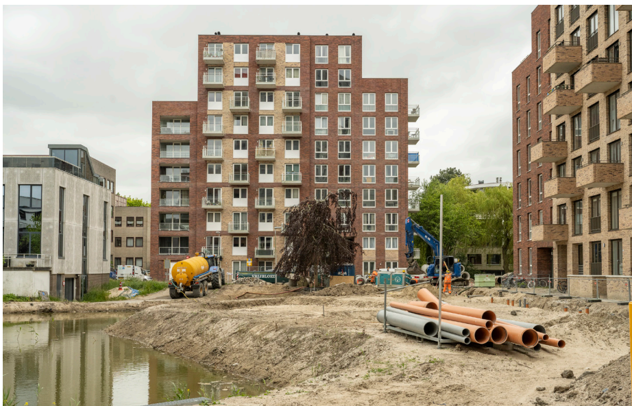
Kanaalpark under construction
